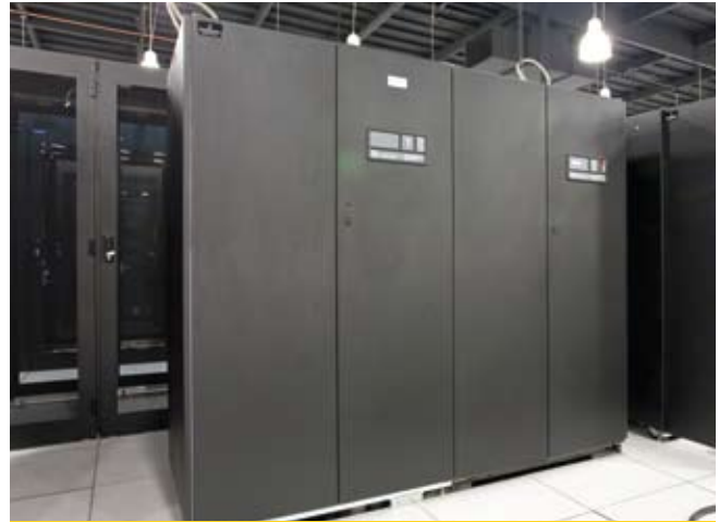
Liebert PPCs with standard TP-1 transformers provide up to 98.7 percent efficiency.
